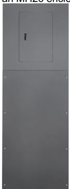
Panel skirt completely installed.
