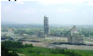
Lafarge Cement manufacturing facility
