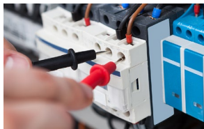
Spain: electrical installations for families in need
